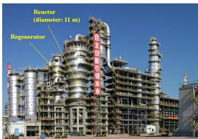
Figure 19. DMTO commercial unit in Shenhua Baotou.
